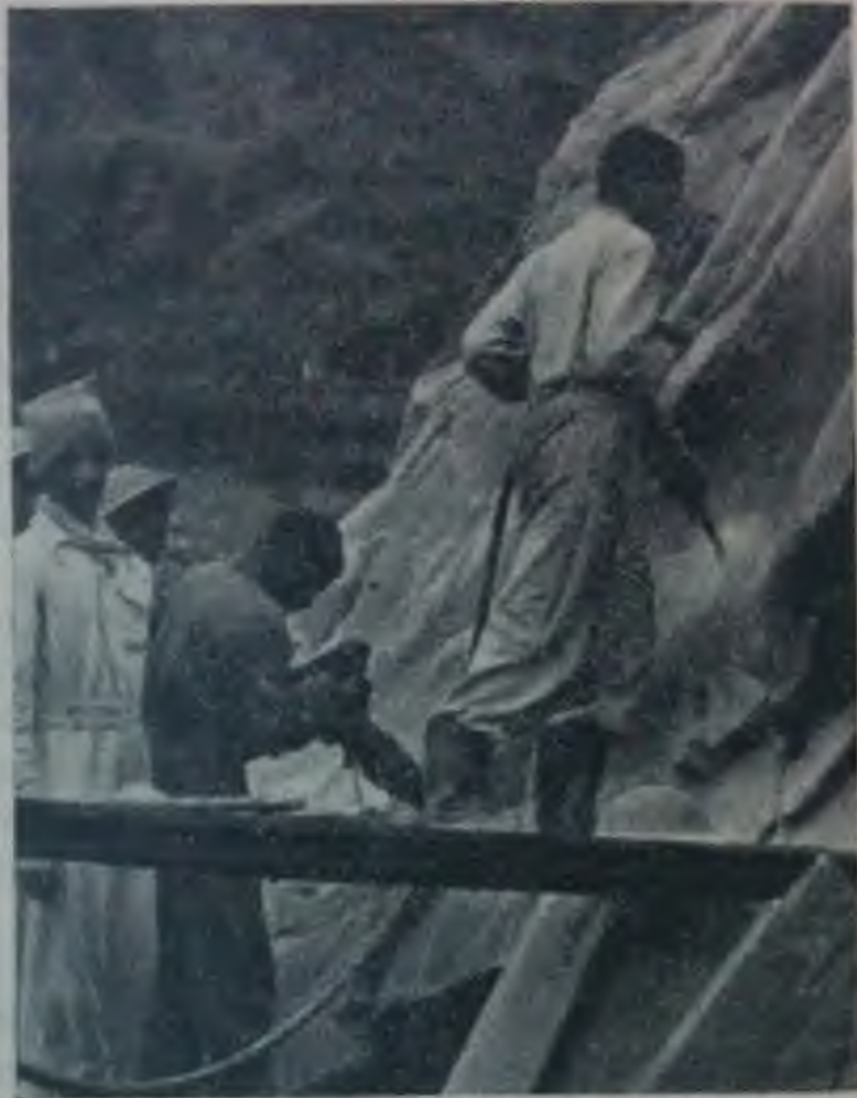
Indian Army engineers blasting a rock to widen the Jammu-Srinagar road.
